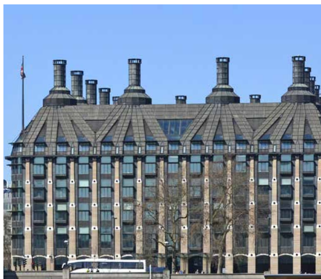
Figure 4 – Nickel aluminium bronze roof, Portcullis House
